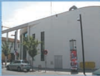
Centre Cultural de Ripollet.
